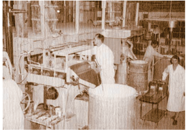
Surrey paint factory at the east end of the Roller Rink. Helmut Much is the paint maker operating the three-roll mill.
