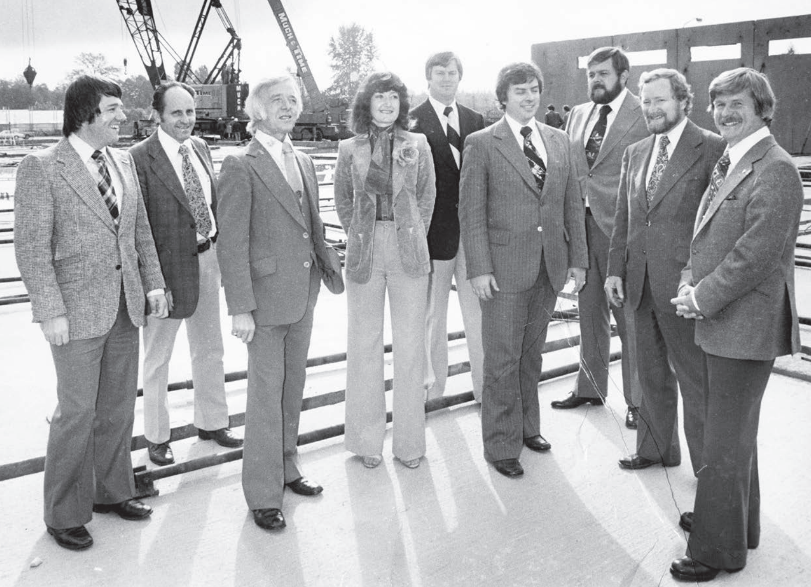
At 6200 Lougheed Highway, Burnaby, construction of a tilt-up building; Dan Treleavan, contractor, Burnaby mayor, banker, Al Mordy, Jim Jackson of BCDC, Burnaby employee, realtor John Williams and Wink Vogel.
